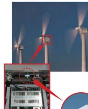
Freeze protection for the control tower of aerogenerator
